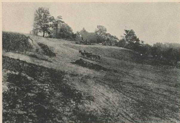
THE 16TH HOLE UNDER CONSTRUCTION One of the very finest holes
